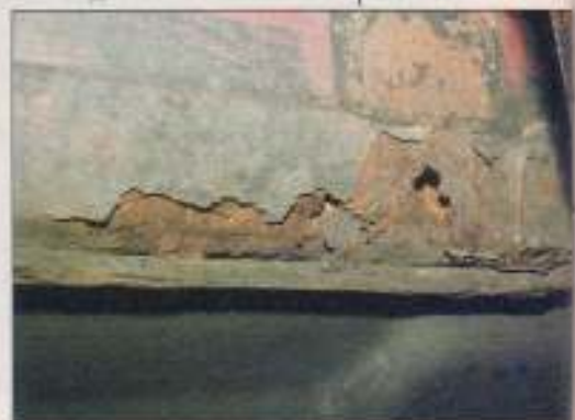
Sills are often weak, and the lower edges are especially vulnerable. If you are looking at a mixture of holes, rusty steel and various patches, bargain on extensive repairs further in!
